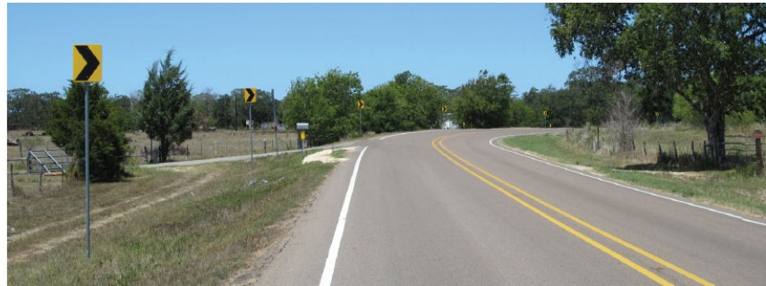
Figure 51. White edge lines, centerline RPMs, and chevrons on a horizontal curve
